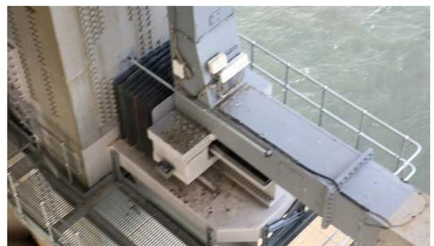
Figure 3. Completed solution, with new bearing installed and supporting the deck truss. One end of the bearing’s T-beam, at the tower, is enclosed in a protective expanding/contracting shroud
