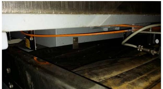
Figure 5. Following installation, connection of a bearing's integrated sensors to the bridge's existing SHM system by means of suitable cabling
