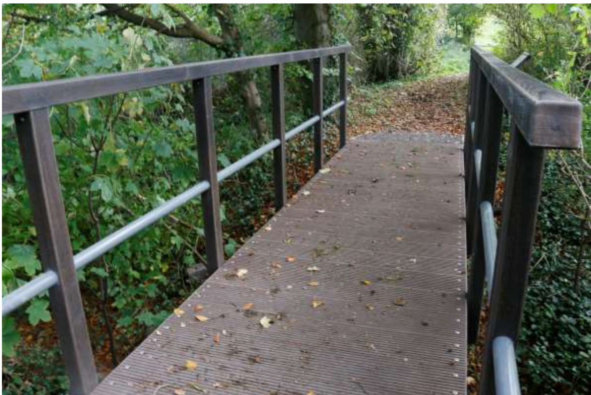
Completed bridge in Dorset showing timber deck effect post s and handrails and castellated planks
