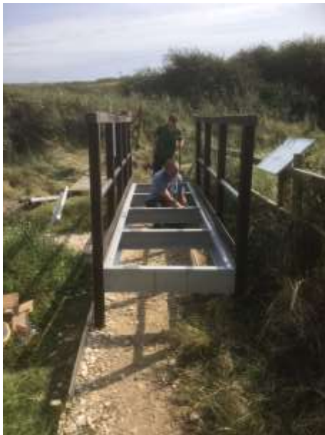
Polybridge being constructed on site in South Gloucestershire
